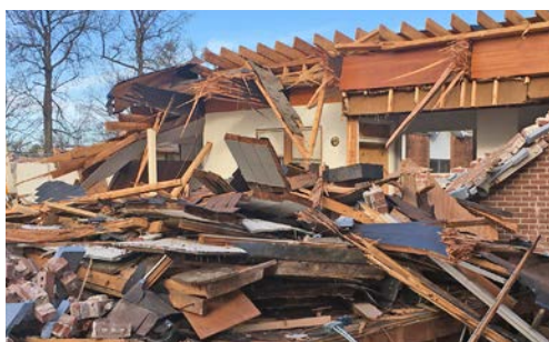
Demolition work is underway at CTK, Memphis.
