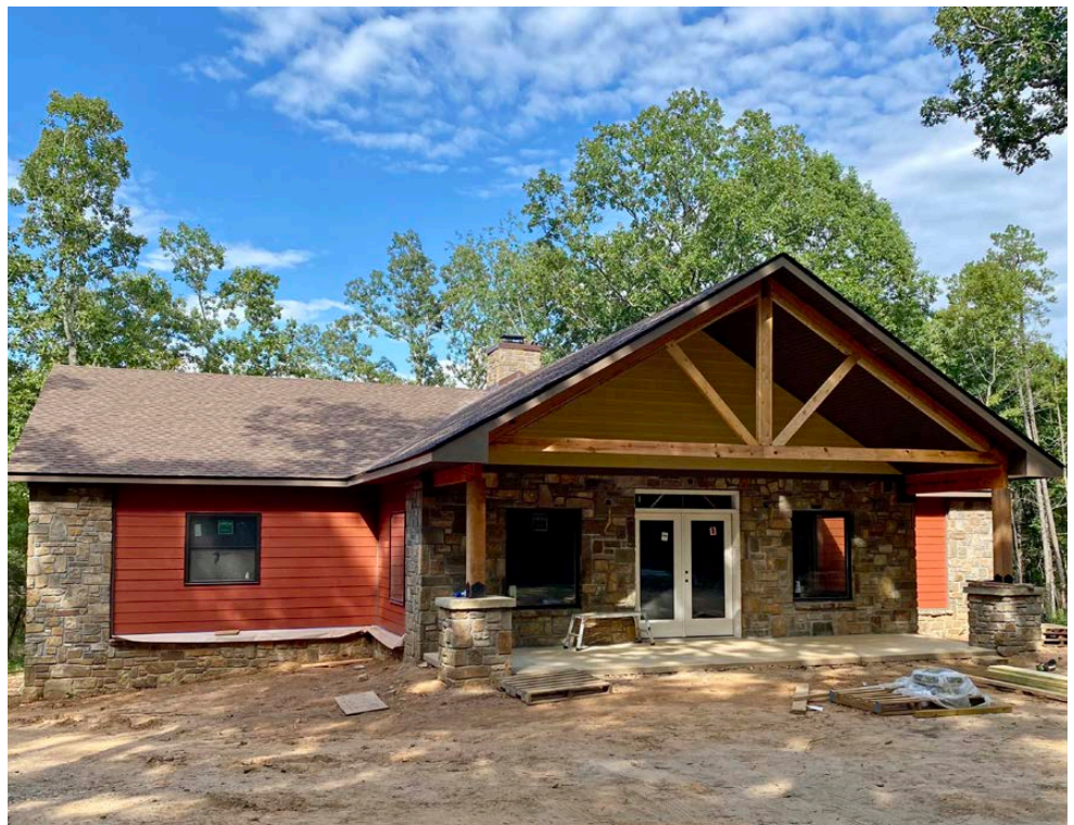
The retreat lodge at Camp Trinity was nearing completion when this photo was taken in August.
